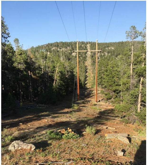
Clean right of way. (Sub-transmission line between Crescent & Lincoln Hills substations)
